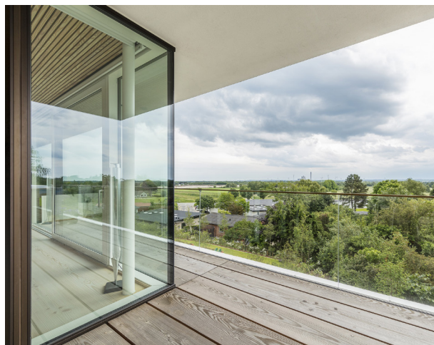
SPECIAL SOLUTION // GLASS TO GLASS CORNER
