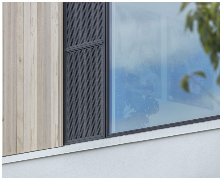
SPECIAL SOLUTION // NATURAL VENTILATION
